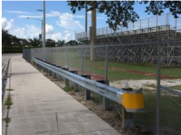
21 - new guardrail installed
